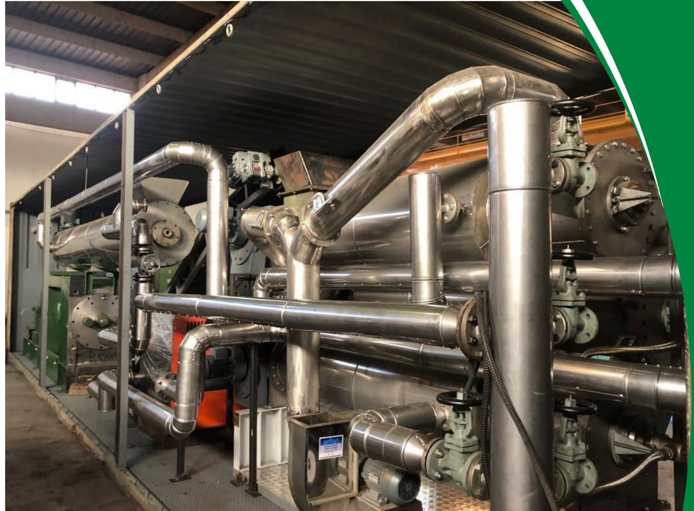
*This container houses the radiant heat processor which eliminates pathogens and eliminates odor. Next, the press will remove the liquid and transfer fluids to the filtration system.*
